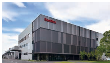
Shiga Plant (Power supplies)
